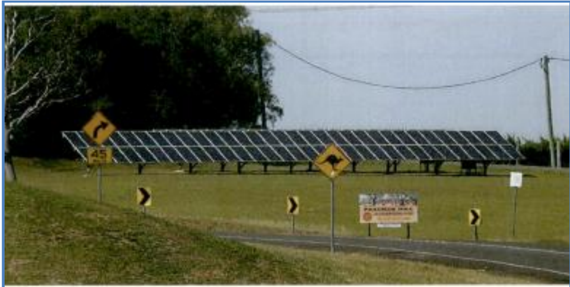
Figure 4: Existing solar energy system at 'Peacock Hill'.
